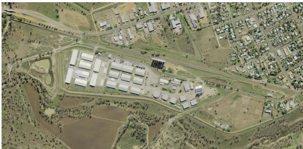
Figure 53: Wee Waa intermodal freight facility
