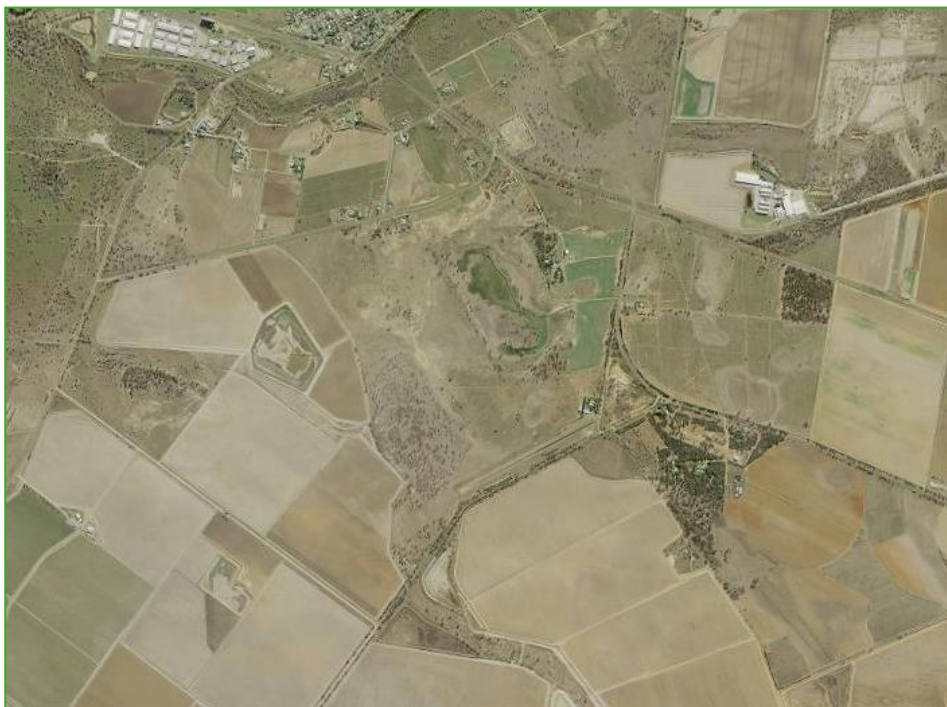
Figure 68: Wee Waa south aerial view of R5 zone
