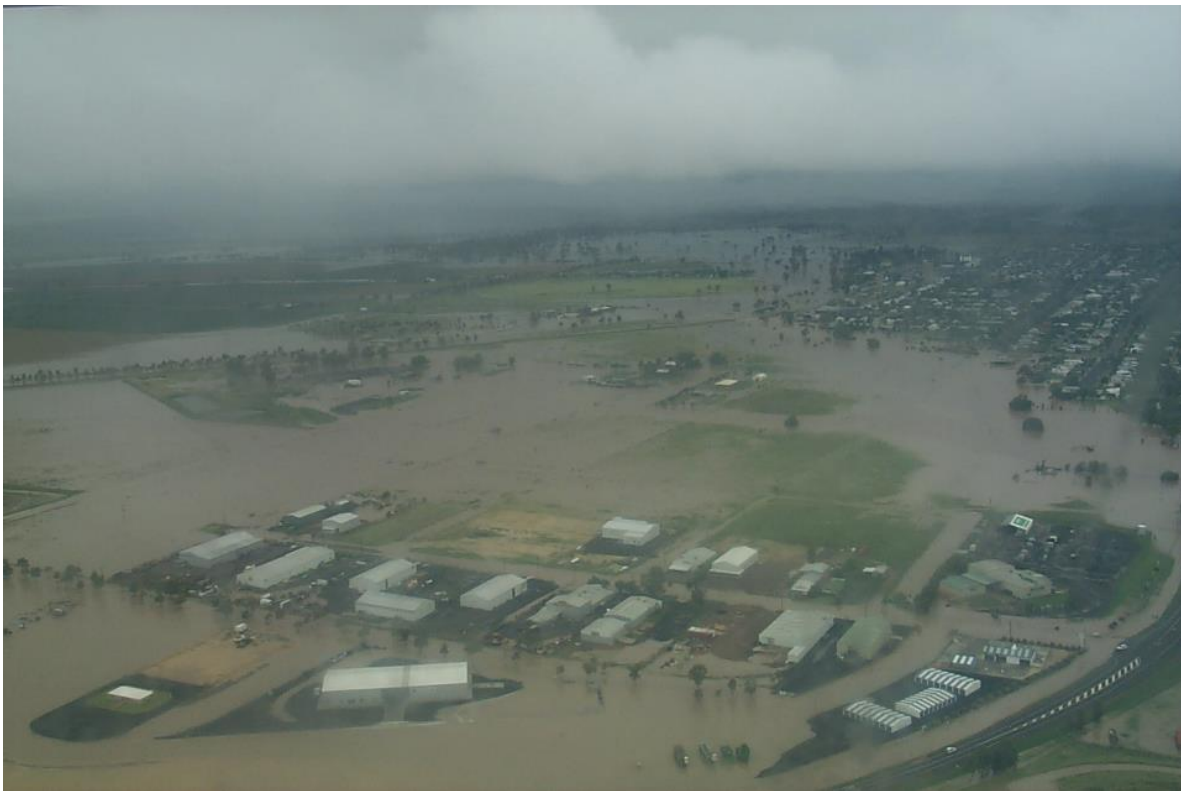
Figure 4.3 - Mulgate Creek flooding, looking east at Francis Street Industrial Estate, December 2004
